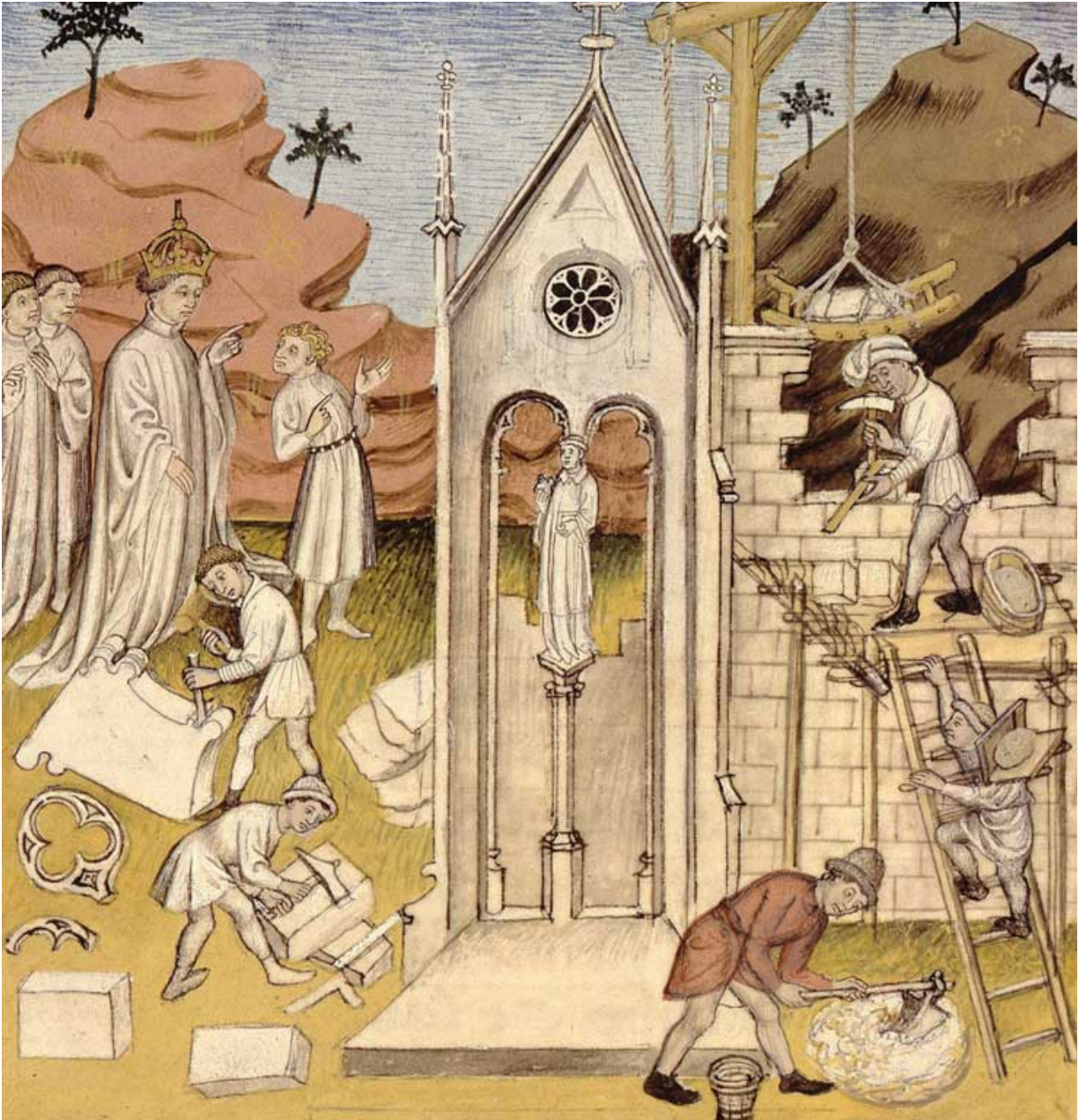
BUILDING A CATHEDRAL
