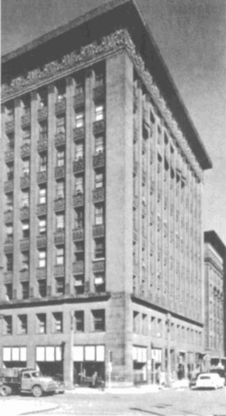
SULLIVAN Wainwright Building, St Louis 1890-1891
